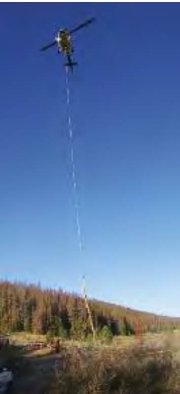
Contract heli-logging doesn’t come cheap, but is necessary in some of the less accessible right-of-way wilderness areas like this one shown in Mountain Parks Electric’s service territory. Photo by Les Shankland.
